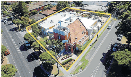
The facilities are mostly in Melbourne's east, including Hughesdale (above).
